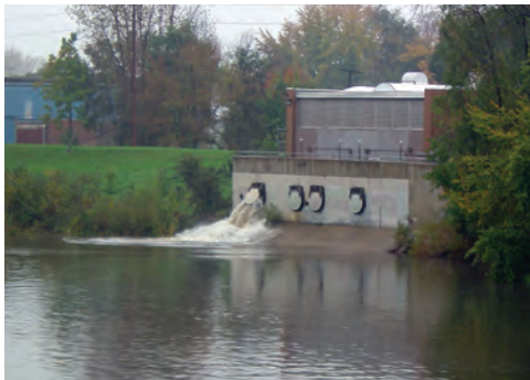
Over the next 20 years, City Utilities will make significant investments to reduce CSOs. The 3rd Street pump station located on the St. Mary's River near Downtown Fort Wayne discharges combined sewage and storm water during heavy rains. Photo: City of Fort Wayne Utilities.
